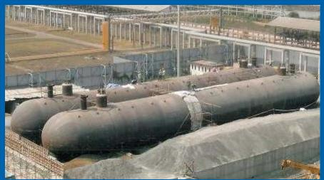
Introduction :-We Manufacturer, Supplier & Exporter of LPG Mounded Bullets. LPG mounded bullets Volumes are from 500 M3 to 20000 M3 Total Storage, as well as Refrigerated mounded for propane storage. Mounded The Bullets designed as per ASME Sec. VIII Div.1, ASME Sec. VIII Div.2 and BS 5500 codes. We have executed facility including storage Mechanical, Civil, Piping, Instrumentation and Electrical.
